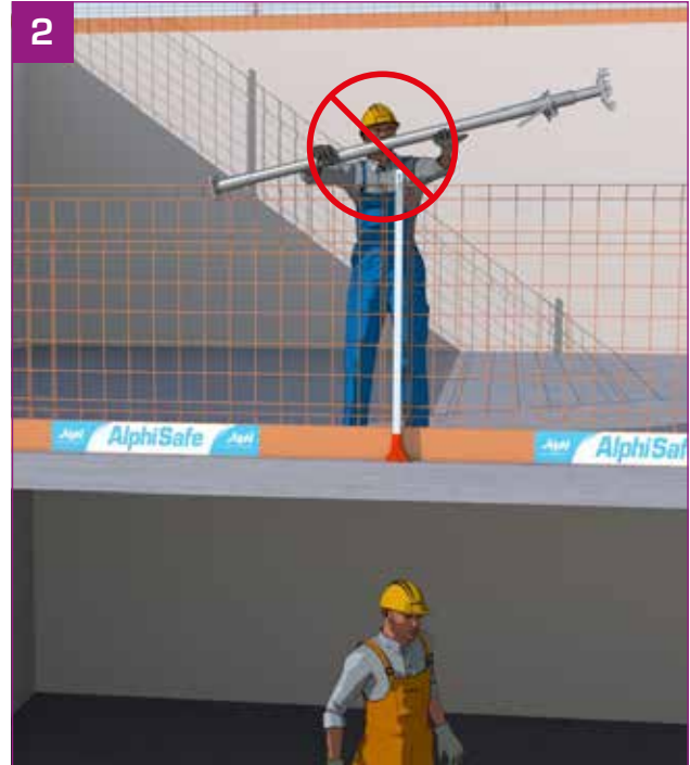
- Do not throw props. Stow them in the suitable racks and move them using a crane.
